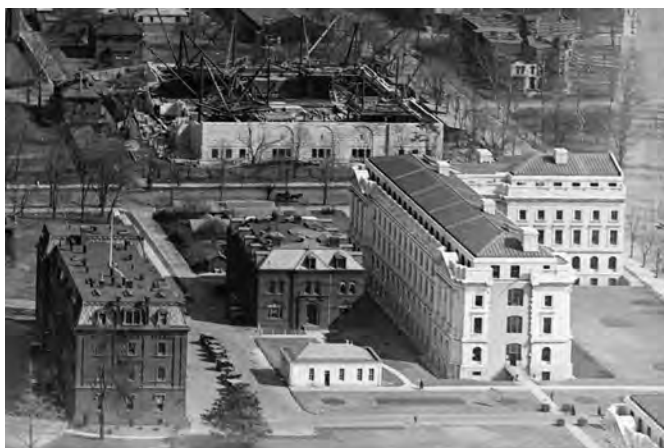
Figure 17. View looking east towards the newly finished East Laboratory (left), Seed Building (center), and Agriculture Building (right). This photograph was taken about 1916. The unfinished building in the background is the Smithsonian's Freer Gallery of Art (author's collection).
